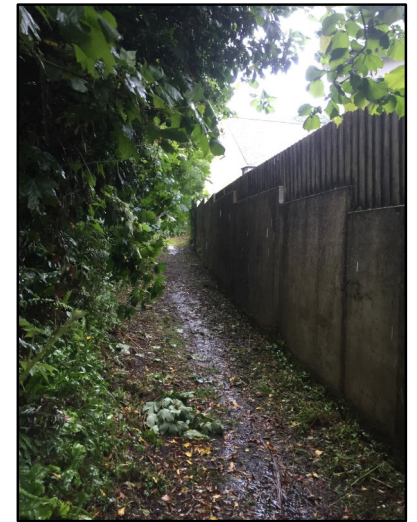
Right: Unsightly bridle path that could transfer into the top of the new site
