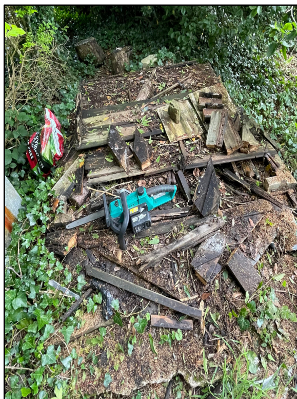
Left: Base layers of the shed being reduced and removed, or good boards stacked to dry out
