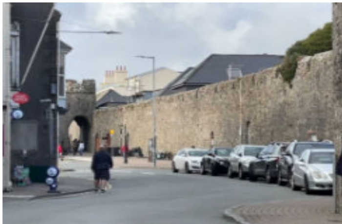
Recent buildings too close and high for the town walls
